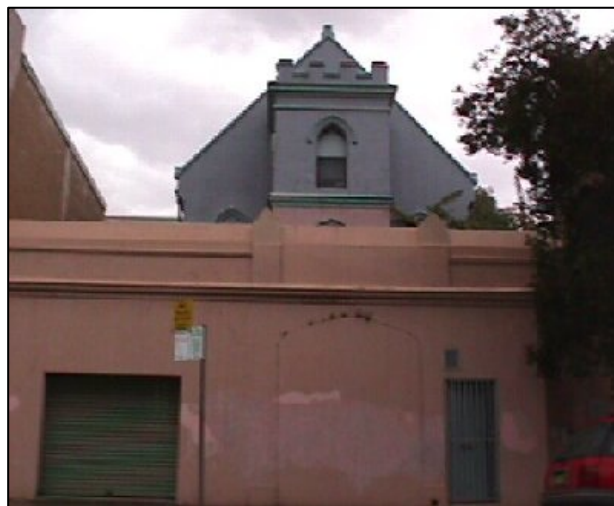
Remains of the old St Michael's Melkite Church in Wellington Street, Redfern. The deconsecrated church building is now part of a housing complex.
